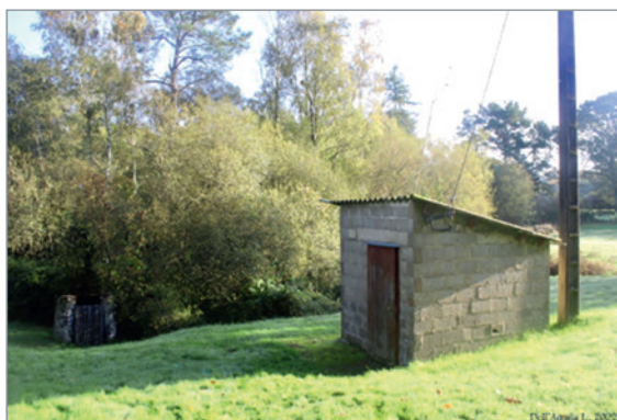
Photo 1 – Station de captage d'un service associatif (Loire-Atlantique). © L. Dell'Aquila – 2022.
