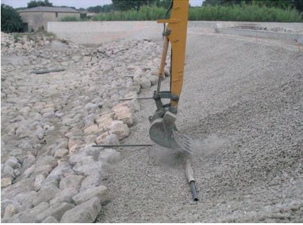
**Photo 5.7.** Comps spillway, installation of outlet drains. (Source: CNR)
