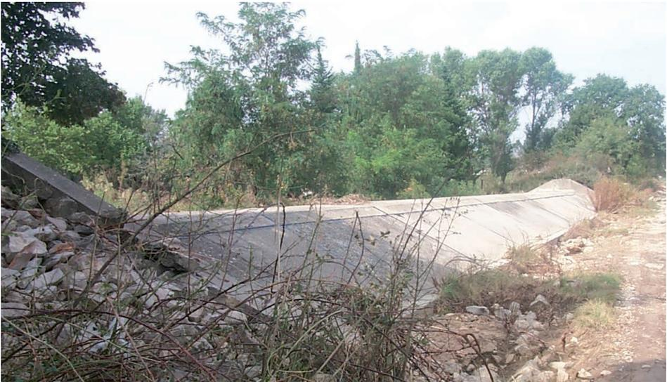
**Photo 1.7.** One of ten Pitot spillways on the left bank of the Vidourle River (after the flood of 2002 and before the levee was reinforced). The Vidourle is to the left. This spillway was renovated in the 20th century (concrete slabs). (Photo: Gérard Degoutte)
