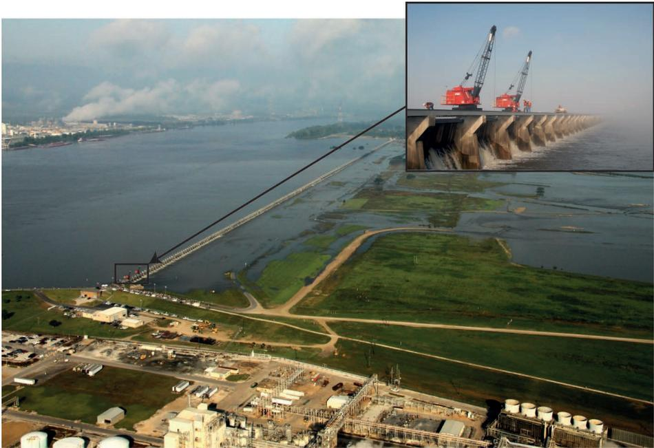
Photo 1.12. Aerial view of the Bonnet-Carré spillway in operation, on the left bank of the Mississippi River. The sticker shows the machine used to move the wooden needles. (Courtesy of US Army Corps of Engineers, public domain)
