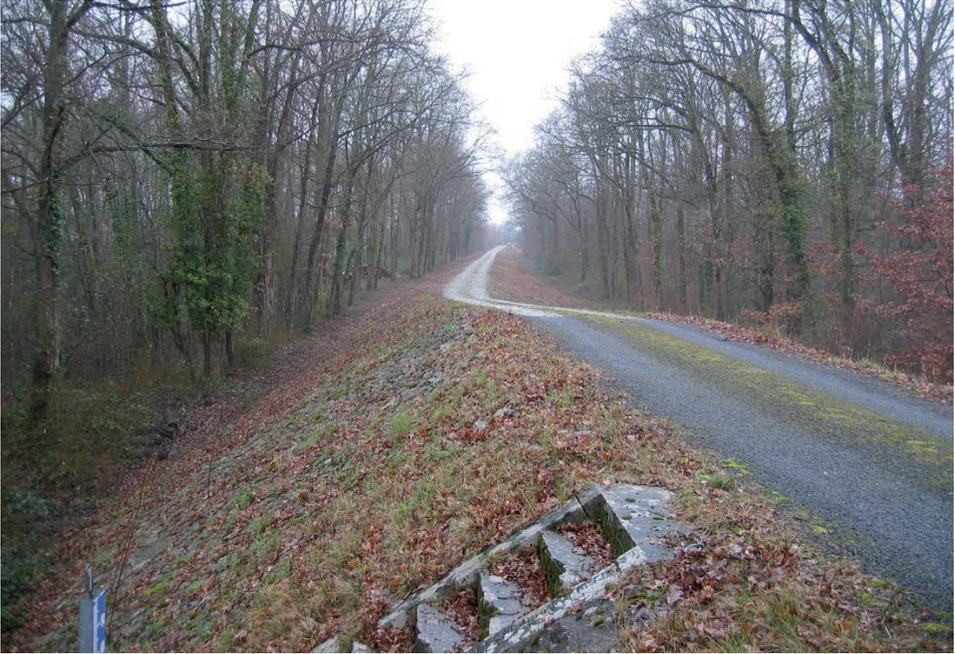
**Photo 1.6.** The Dampierre Spillway on the left bank of the Loire River, without a fuse plug. The hydraulic function of this structure is not apparent. (Photo: DREAL Centre)
