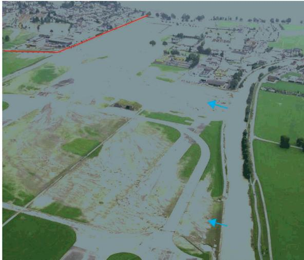
**Photo 5.19.** Aa Engelberg River at its junction with Constance Lake in 2005. We can see two of the three spillways in operation. A secondary levee is under construction to protect inhabited areas (red line). (Photo: the Swiss Air Force in Rosier, 2005)
