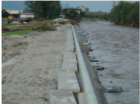
**Photo 5.18.** Fuse plug slabs after the 2005 flood. (Source: Hunzinger, 2007)
