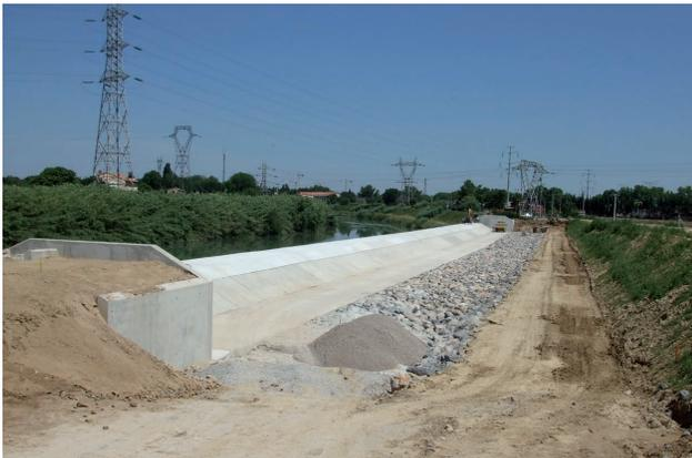
**Photo 1.11.** The so-called diverter spillway in Lattes on the left bank of the Lez River, under construction. This 150-m-long spillway diverts floodwater towards a channel (see Figure 1.11). (Photo: BRL-i)
