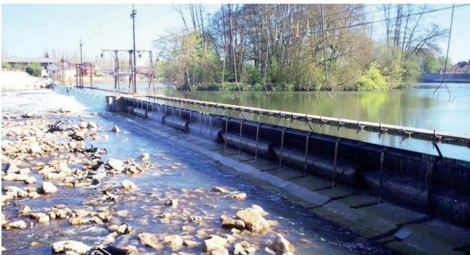
**Photo 5.13.** Auxonne movable dam with 1.3-m-high gates. (Source: BRL-i)
