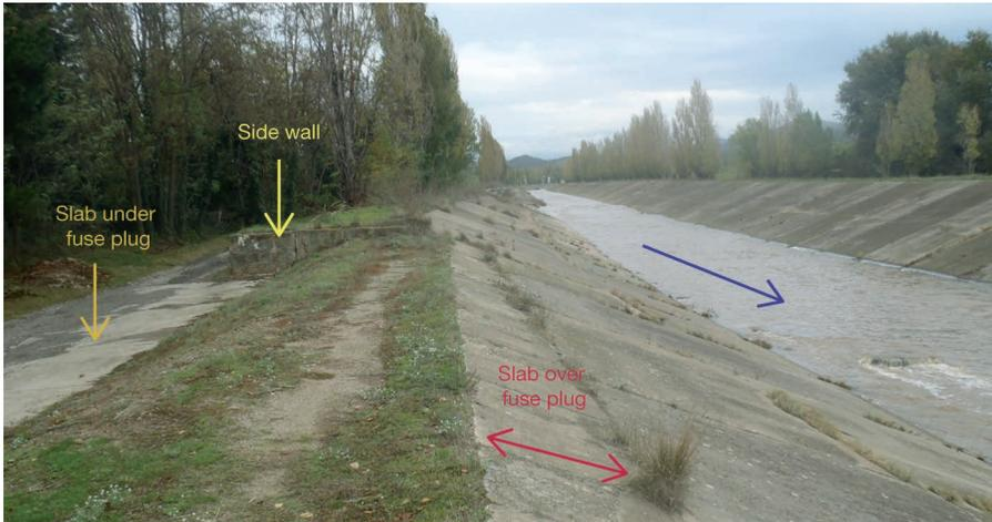
**Photo 5.16.** Reyran fuse plug spillway (Var department). (Photo G. Degoutte)
