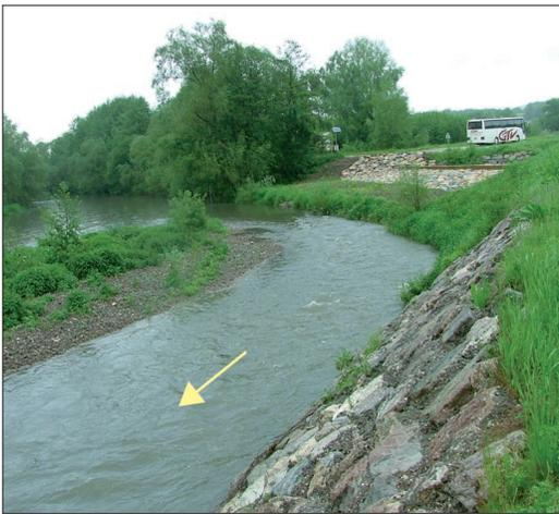
**Photo 4.4** Spillway on the left bank of the Savoureuse River (built by the Pays de Montbéliard Urban Community). The spillway's placement on a concave bank helps preserve a channel between the deposits and the spillway. Vegetation must not be allowed to form on the island that is created.
