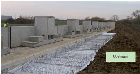
**Photos 5.14 and 5.15.** Fusegates on the Allan River. Top: the gates have been installed; Bottom: the gates are nearing completion with discharging tower and joints between the gates; the Reno mattress is being installed. (Photos: Montbeliard Authorities - CAPM)
