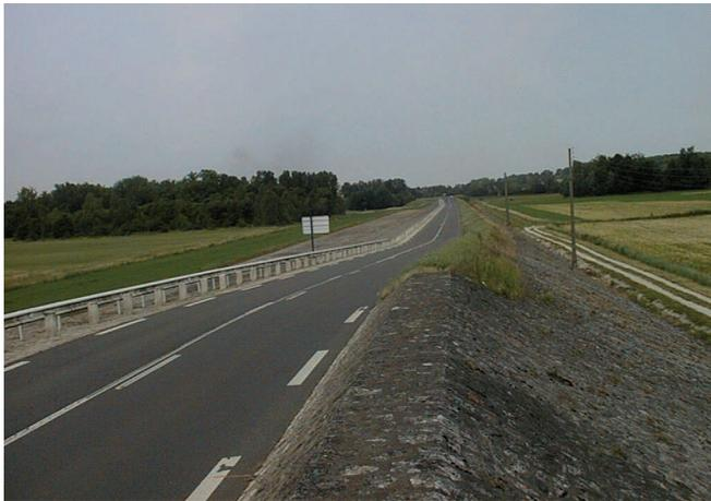
**Photo 1.5.** The Montlivaut spillway on the left bank of the Loire River, which spills floodwater into the upstream part of the Blois leveed area. It was built just like the Jargeau spillway but is covered by a road and located at the site of a breach caused by the 1846 flood. (Source: Gérard Degoutte)
