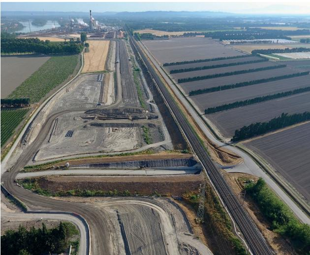
**Photo 5.2.** Aerial view of the duckbill-shaped earthen embankment built along an underpass on the Arles-Tarascon railway. (Photo: SYMADREM)
