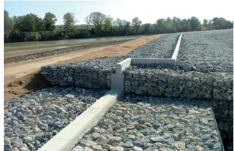
**Photos 5.11 and 5.12.** Lunel spillway on the Vidourle River. On the riverside (on the right in the left-hand picture and on the left in the right-hand picture), the Reno mattress is covered in canvas before sodding. On the right, detail of a notched section. Note the concrete beam embedded in the levee to serve as a weir. (Source: Gérard Degoutte)
