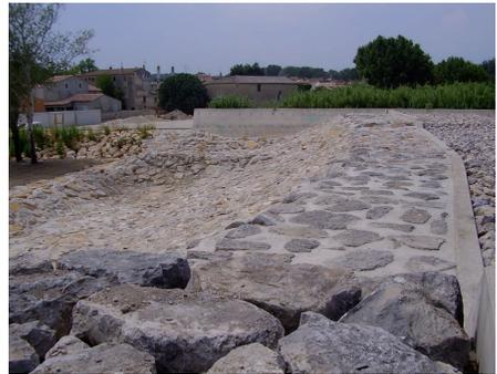
**Photo 5.10.** Downstream face and completed stilling basin. (Source: CNR)
