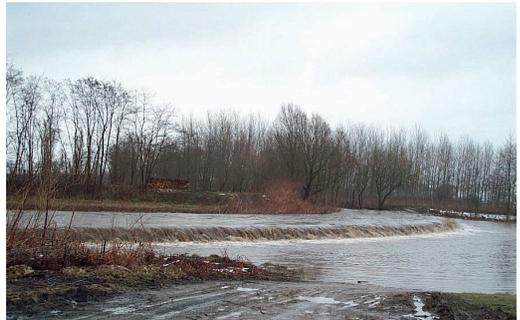
**Photos 1.9 and 1.10.** Masonry spillway on the right bank of the Giessen River (Bas-Rhin), around 90 m long. (Photos: Bas-Rhin DDT)
