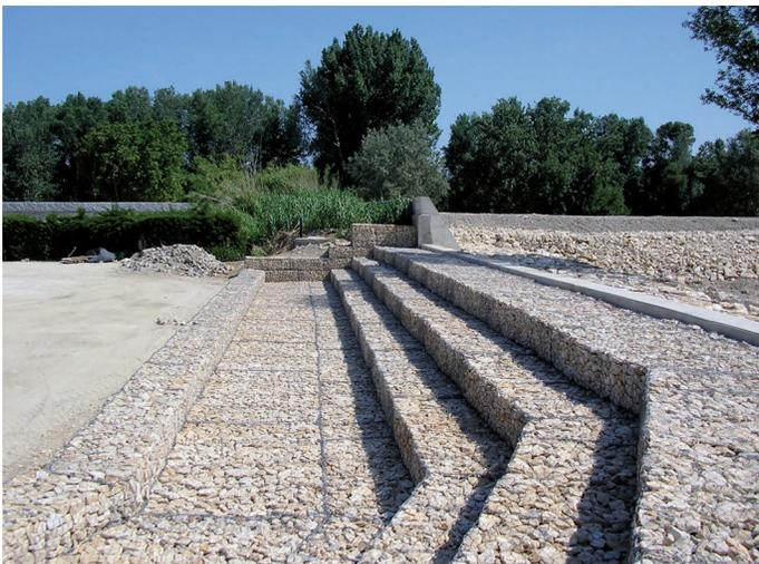
**Photo 5.1.** Comps spillway (Gard department) with the downstream face made of gabions. (Source: DDT 30)
