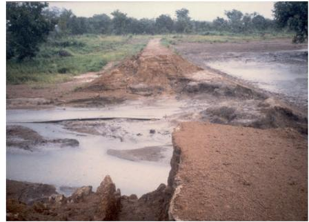
**Photos 1.1 and 1.2.** Overtopping of two small earthen dams of similar construction; of short duration on the left and long duration on the right. On the right, there are stepped shapes. Though they are not levees, the mechanism is the same. (Photos: Paul Royet, 1983)
