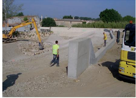
**Photo 5.8.** The crest beam formwork has been stripped off. (Source: CNR)
