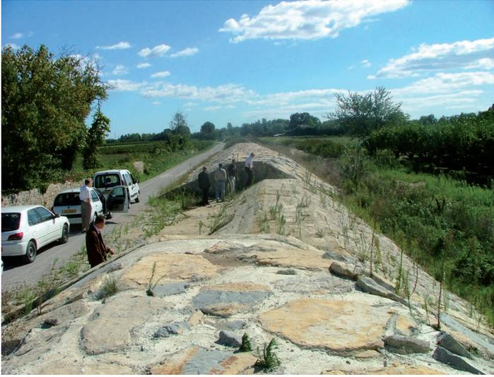
**Photo 1.8.** Another Pitot spillway on the Vidourle after the levee was reinforced following the 2002 flood. The Vidourle is on the right. We can see the vertical sidewall between the spillway and the regular section of the levee. (Photo: Gérard Degoutte)
