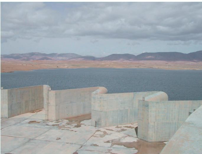
**Photo 5.3.** Labyrinth spillway on the Fontaine des Gazelles dam (Algeria).
