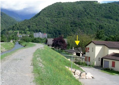
**Photo 4.2** The Doménon River after an emergency repair of the levee, view from downstream. The yellow arrow points to the flooded and alluviated house in the Summer of 2005, also shown in the second photo. (Photo: R. Tourment, INRAE)
