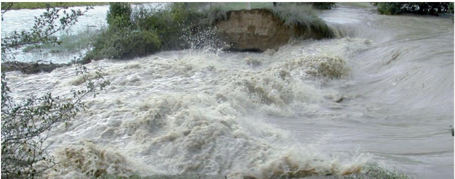
**Photo 1.3.** Breach on the left bank of the Vidourle River in Aimargues on 9 September 2002 (4 m × 25 m, 294 m<sup>3</sup>/s as indicated by SAFEGE modelling for SIIV). In the foreground, the top of a “step” has been cut out. (Photo: Aimargues town hall)
