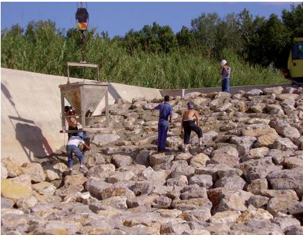
**Photo 5.9.** Placement of downstream riprap. (Source: CNR)
