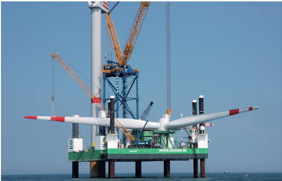
■ Photo 11 : blade (126 m in diameter) being mounted on the mast in the 300 MW Thornton bank offshore wind farm in Belgium (© Deme, BE).
