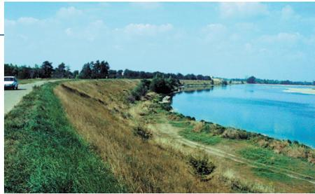
*DIKE: An artificial structure, flood protection embankment or barrier that protects against river flooding, at least a part of which is built above natural ground level. It is designed to periodically contain a high discharge of water and thus protect areas that are naturally prone to flooding. (The term “levee” is often used along the French River Loire in common with certain areas of the USA).*
