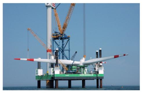
■ Photo 11: blade (126 m in diameter) being mounted on the mast in the 300 MW Thornton bank offshore wind farm in Belgium (© Deme, BE).
